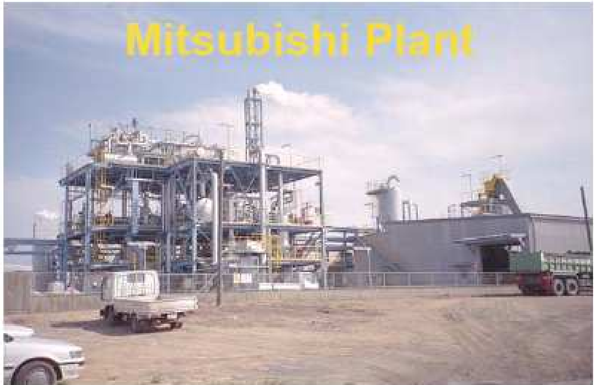
Usine de production de E-fuel www.enertech.com/technology/slurrycarb.html
