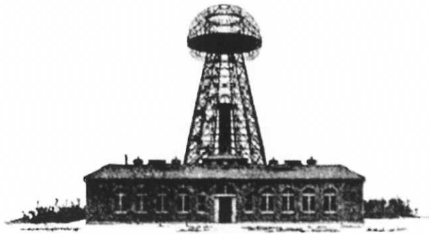
Actual photograph of the Warden-Cliff tower, prior to its demolition in 1917 84
